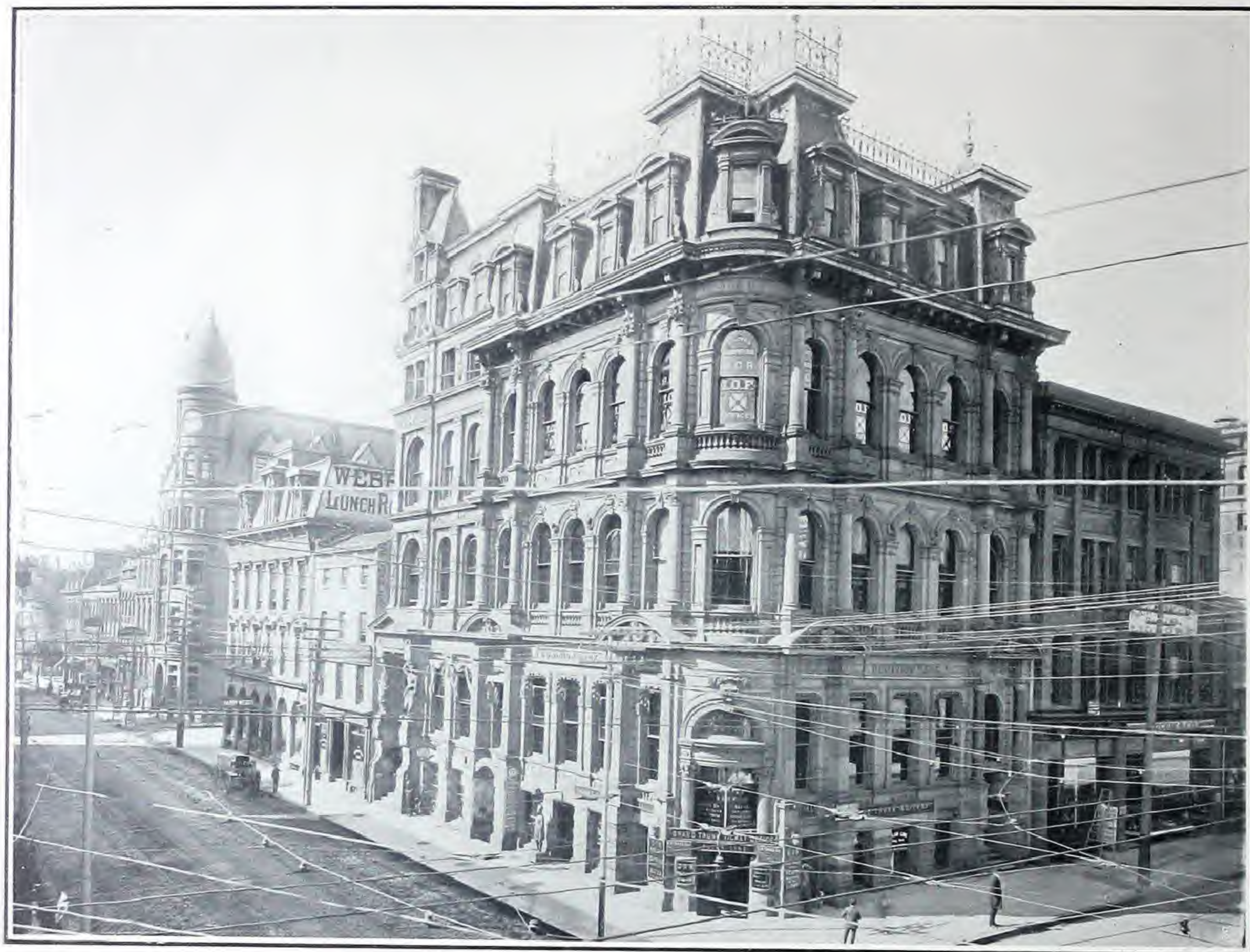
Fig. 192.—Dominion Bank, Toronto, (Head Office) In which the "Hayes" Patent Lathing was used.
